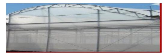
Figure 3: A Polyethylene film covered greenhouse
